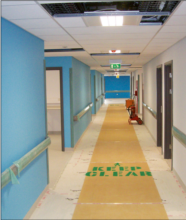
Figure 13a Keep fire exits clearly signed and free from obstructions
