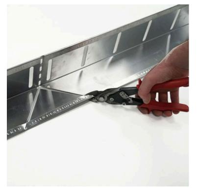
To form a corner, remove the centre 'v piece' with a pair of tin snips. The two sections either side can now be bent to form an internal or external corner as required.
