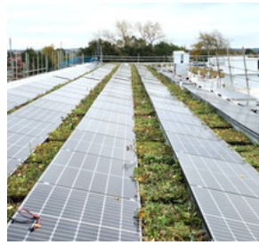
Roofing & Green Roofing
