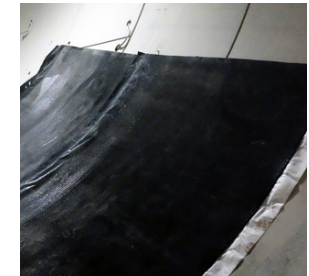
Tunnel & Underground Works
